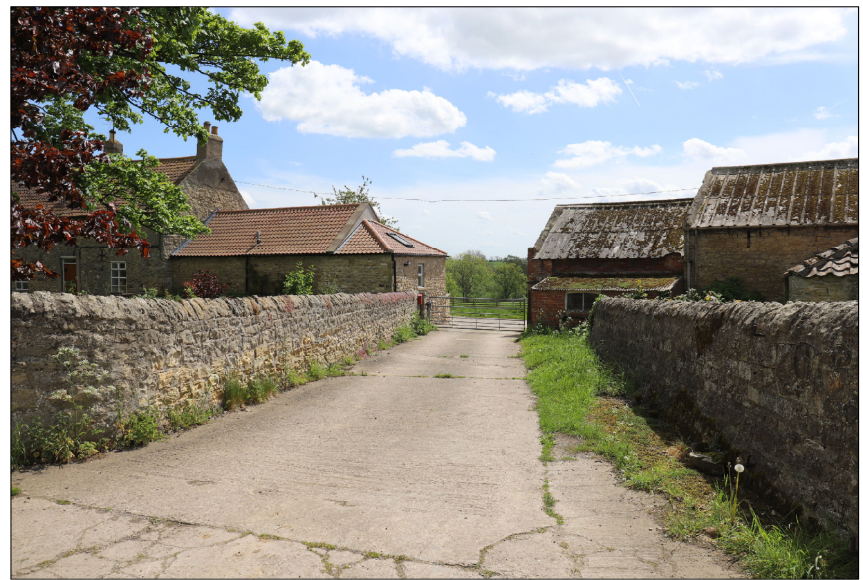
Plate 18) View of proposed cable route between Manor Farmhouse and threshing barn, Brafferton looking south
